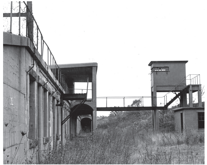
Parade wall of Battery Blair with battery commander's station to the right and plotting room below.
